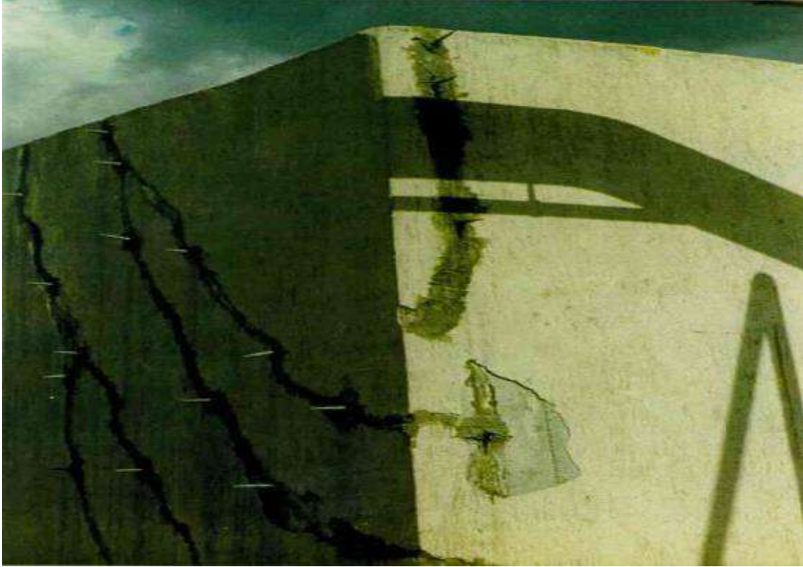
EPOXY İLE STATİK TAKVİYE
