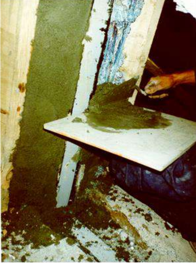
EPOXY REPAIR MORTAR
